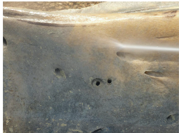
Figure 3. Cleaning tests with pressurized water designed to remove the black dirt under the paint. Image: © MCNB / ICP.
