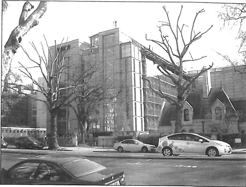
Fig. 2. Darwin Centre Phase 1 from Queens Gate.
