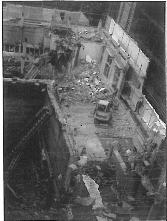
Fig 5. Demolition of the Zoology Spirit Building.
