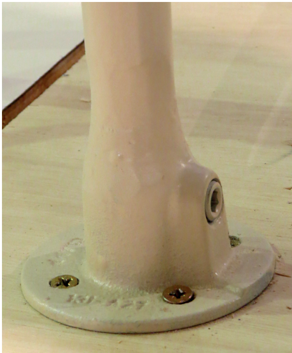
Figure 8. A steel floor plate welded to the bottom of one of the upright steel tubular supports, within which a 22mm diameter threaded bar is welded. This bar runs through the wooden base and is secured underneath with nuts and spring washers. Image: Nigel Larkin.
